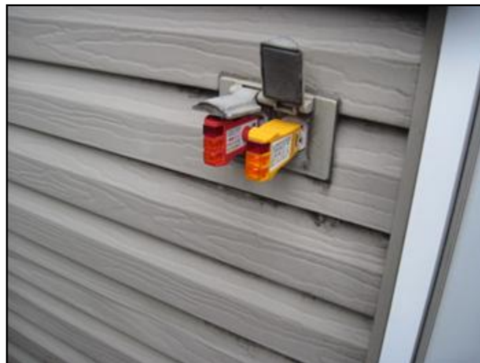
Test indicates absence of protection
