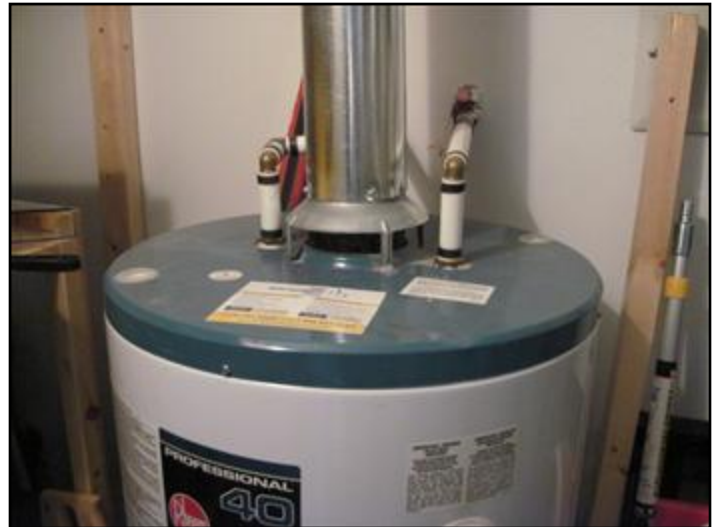
Gas fired water heater in utility room
