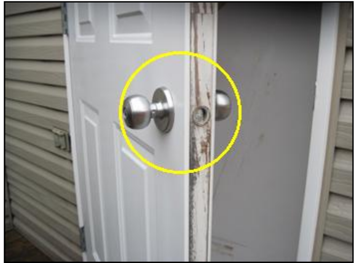
Door latch jammed main floor
