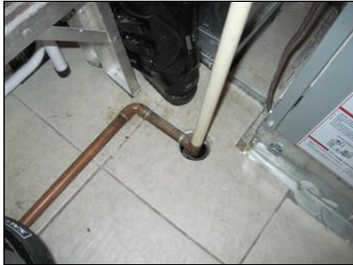
Floor drain installed in utility room
