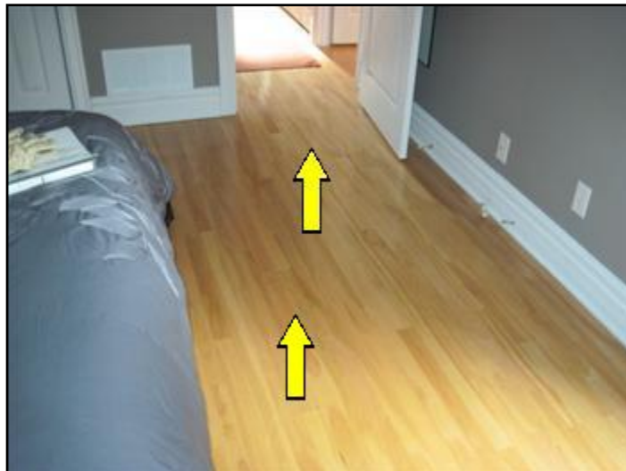
Floor level dips towards hallway
