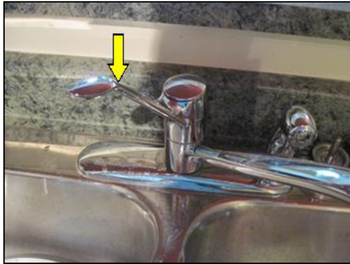
Kitchen faucet handle loose
