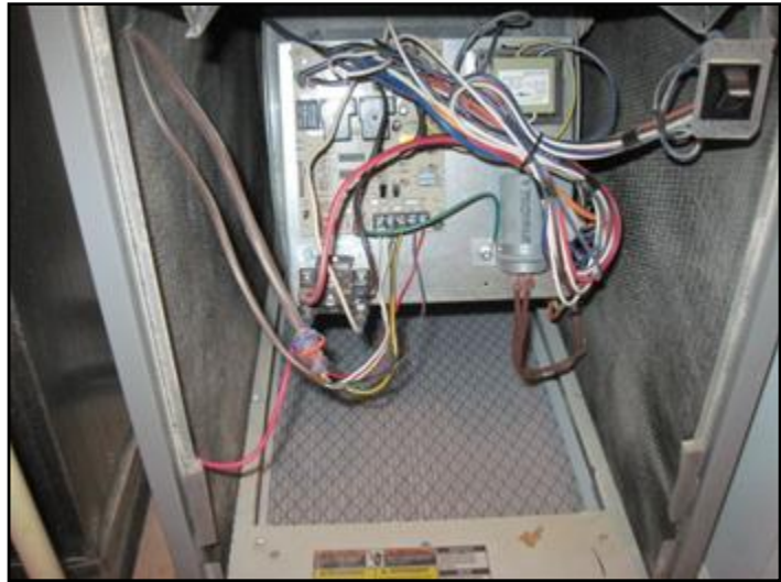
View of air blower and filter chamber
