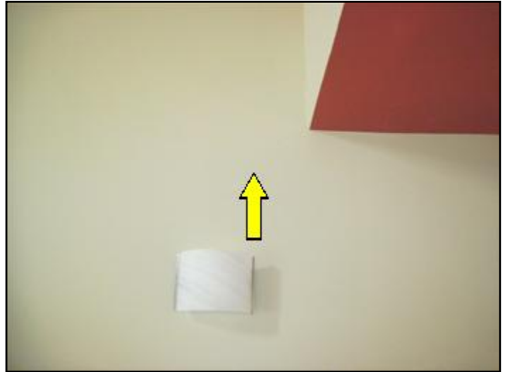
Crack below mezzanine on left wall
