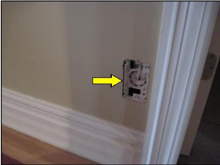
Hose connection for central vac missing cover
