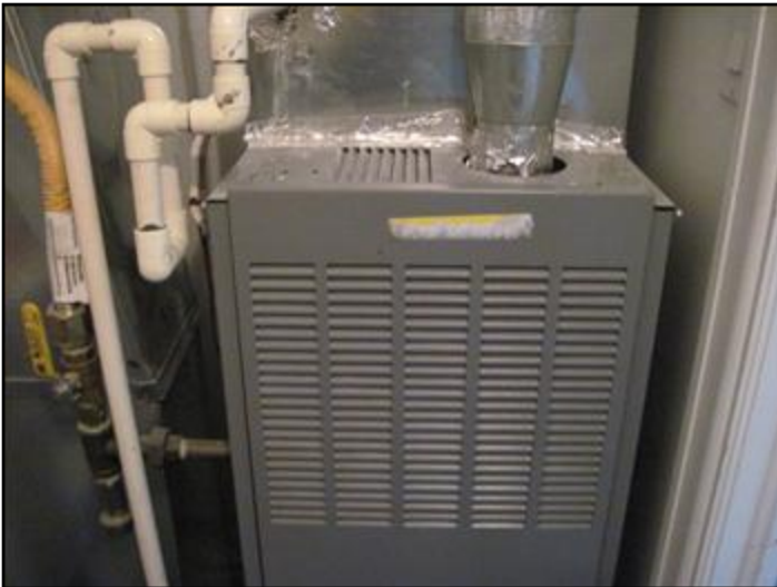
Gas fired forced air furnace
