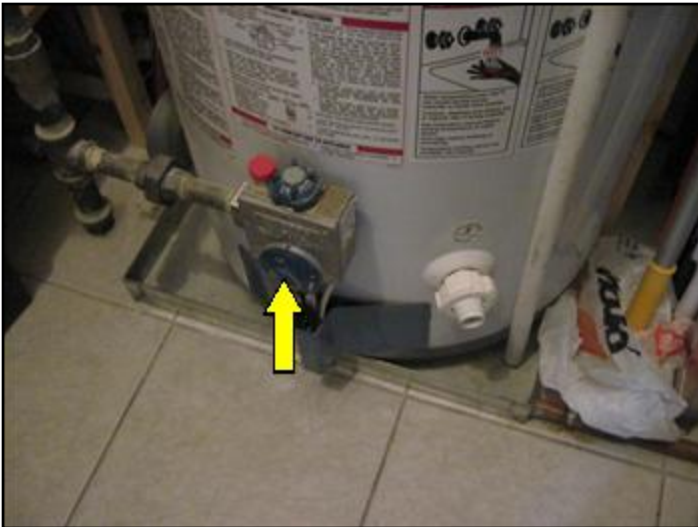
Water heater temperature control
