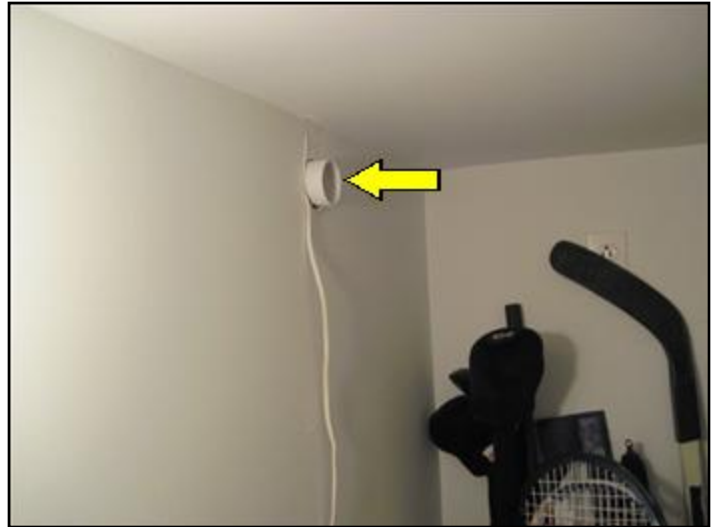
Pipe connection for central vac power unit
