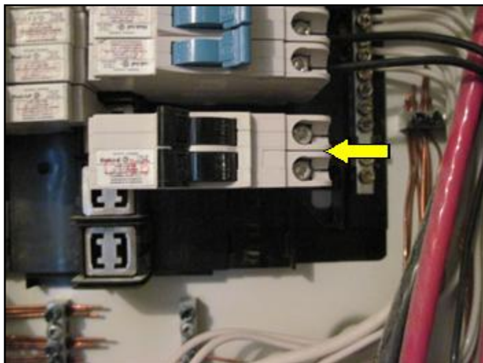
Breaker installed but not in use
