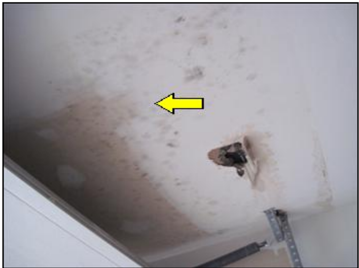
Presence of mould on garage ceiling
