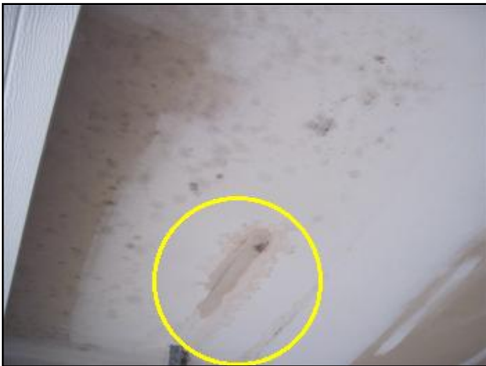
Main water leak in garage ceiling
