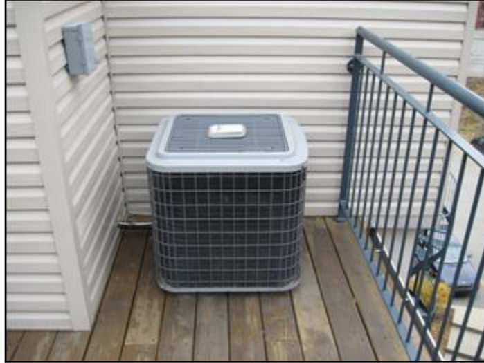
AC condenser unit on rear exterior deck
