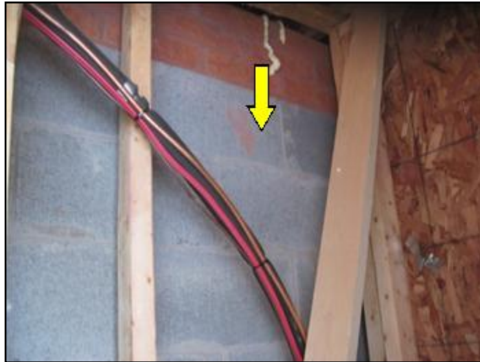
View of concrete block dividing wall
