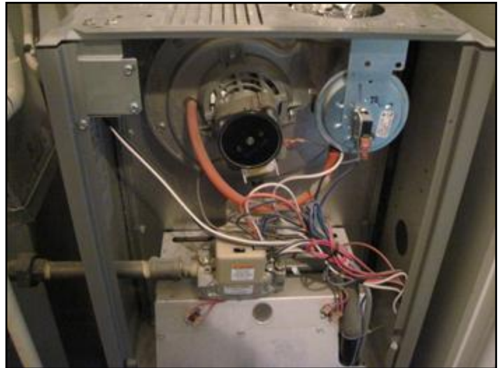
View of blower and burner chamber
