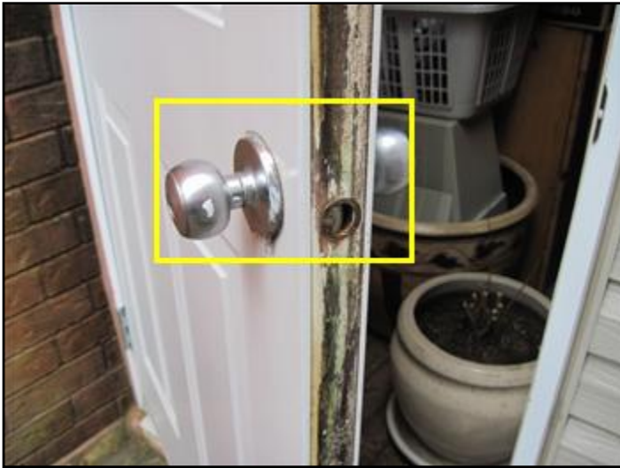
Door latch jammed 2nd floor
