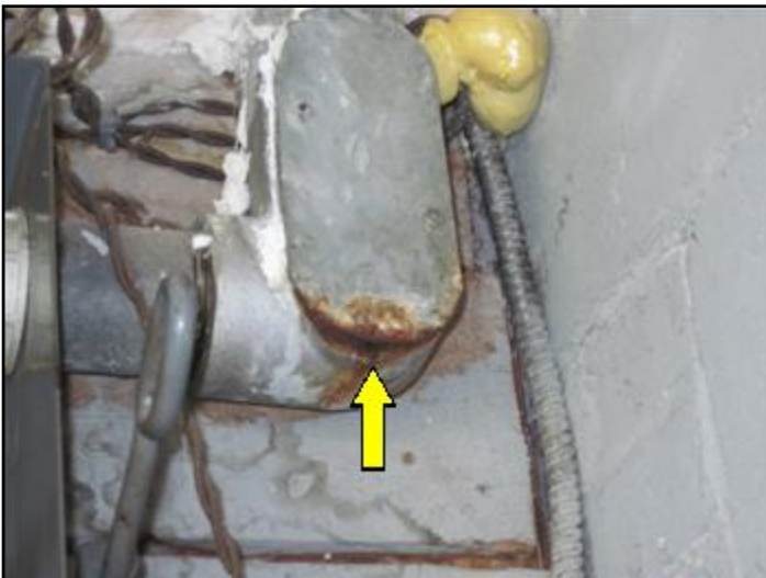
Corrosion at base of electrical conduit
