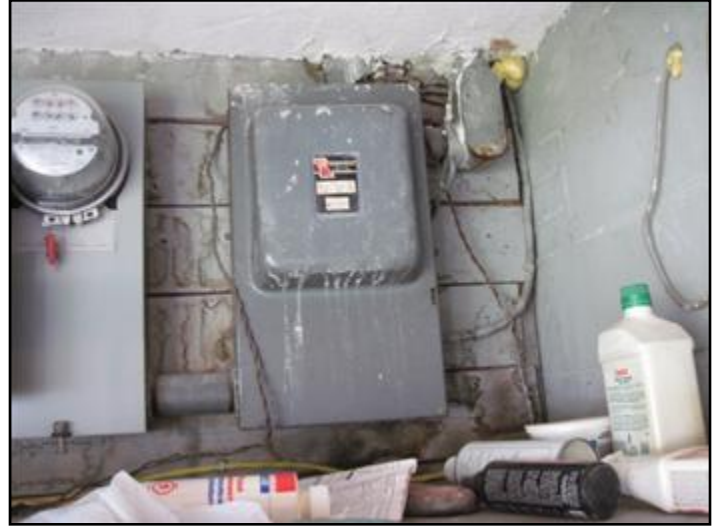
Main electrical disconnect switch
