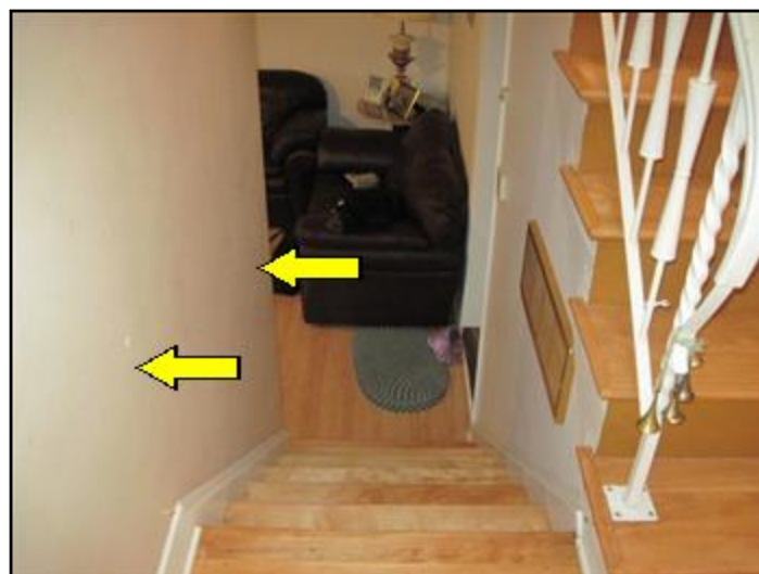
Handrail missing
