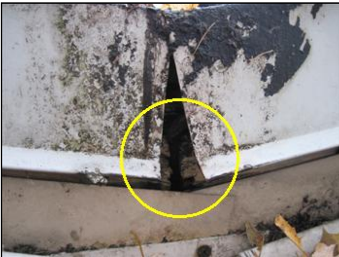
Water penetrating wood exposed
