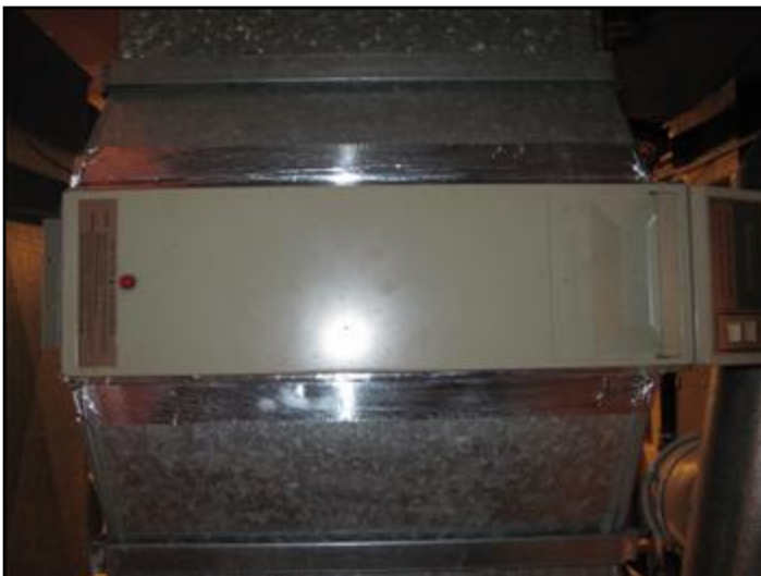
Electronic air filter
