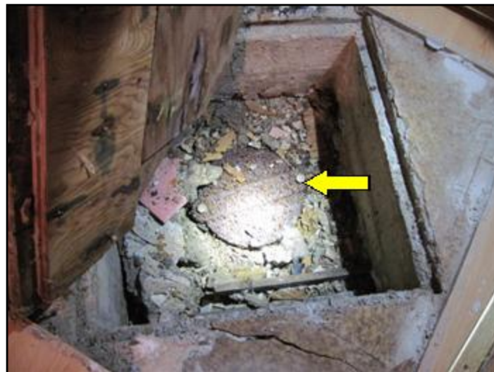
Sewer backflow prevention device
