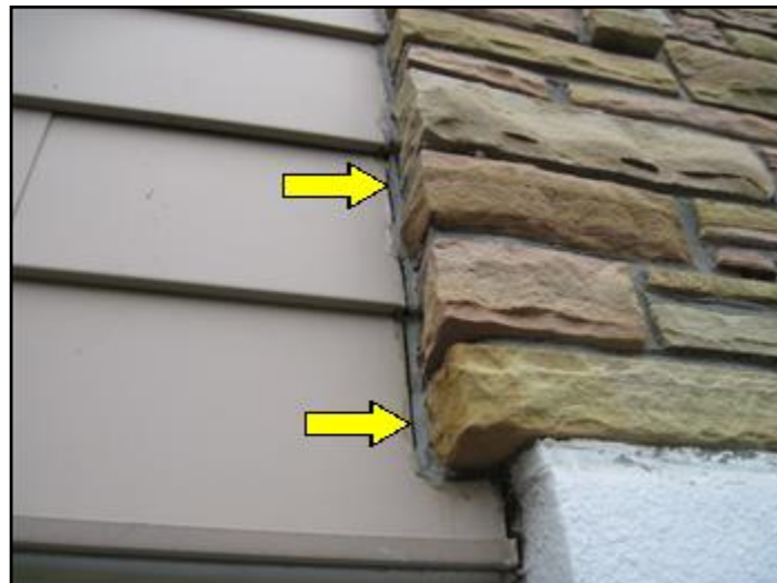
Caulking joint due for replacement front wall
