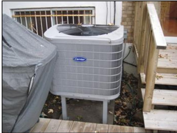
Heat pump condenser unit
