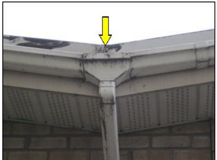
Exposed fascia on rear section
