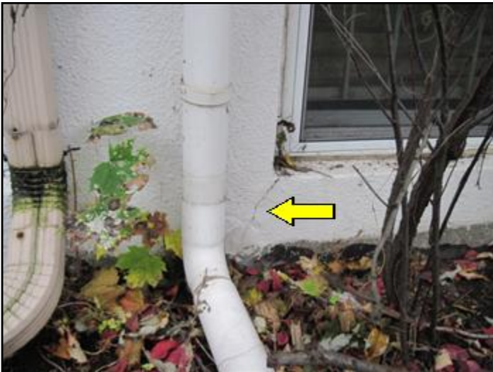
Crack front wall
