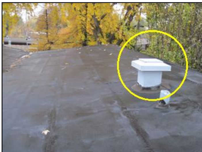
Roof vent on roof surface
