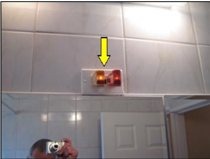
GFI under test failed to trip
