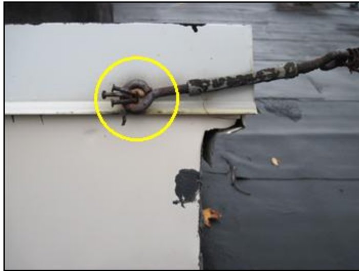
Cable attachment to roof
