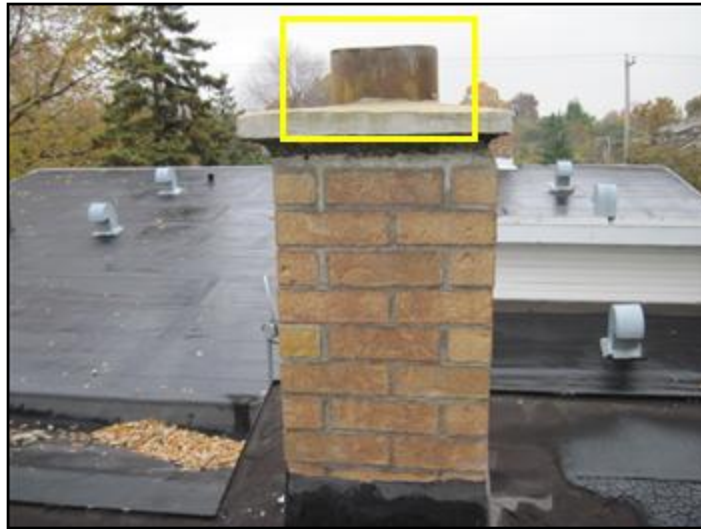
Chimney cap missing
