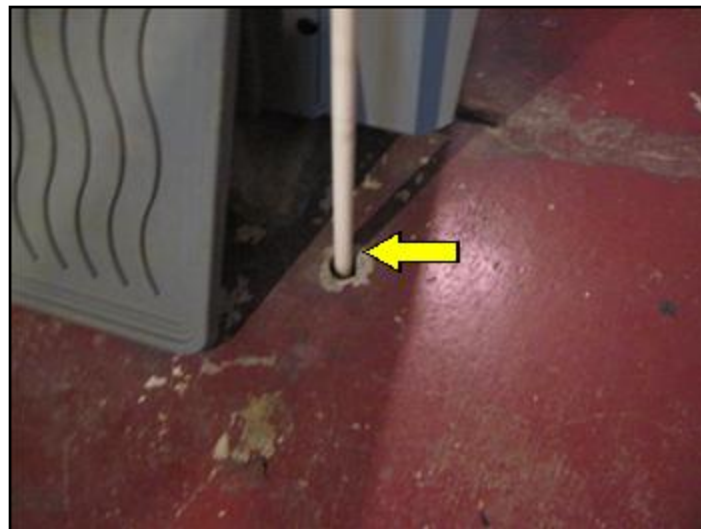
Condensate line discharge point
