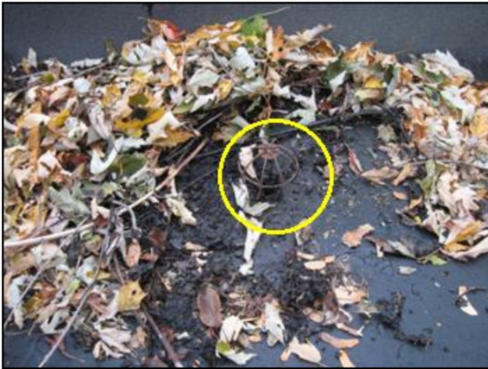
Clogged roof drain
