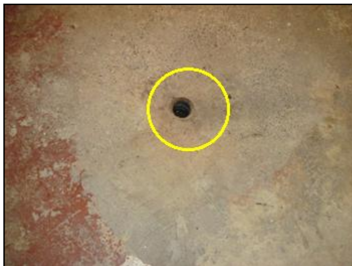
Grate missing on basement floor drain
