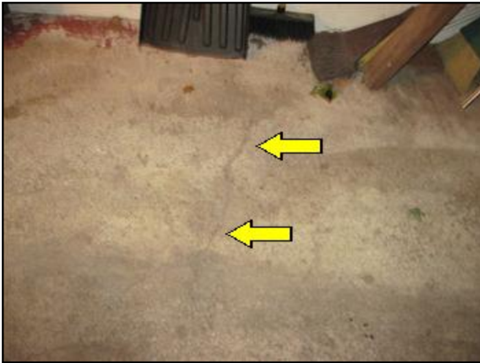
Cracks in garage floor slab
