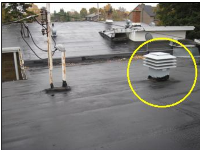
Roof vent on roof surface
