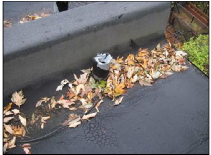
Debris accumulation on roof
