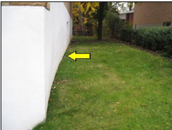
Lot sloping towards foundation on right side
