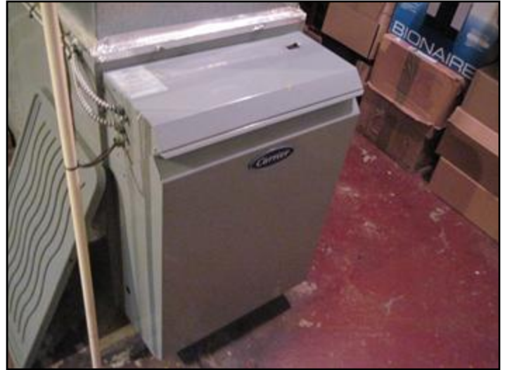
Carrier forced air furnace
