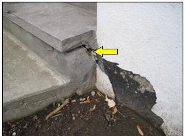
Settlement has caused a gap to open
