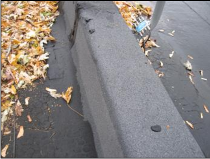
View of membrane without coating
