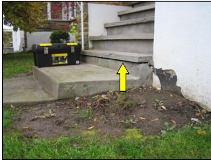
Settlement has caused a gap to open
