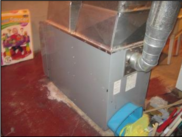
Carrier forced air furnace
